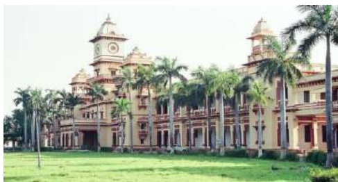
Department of Electrical Engineering
